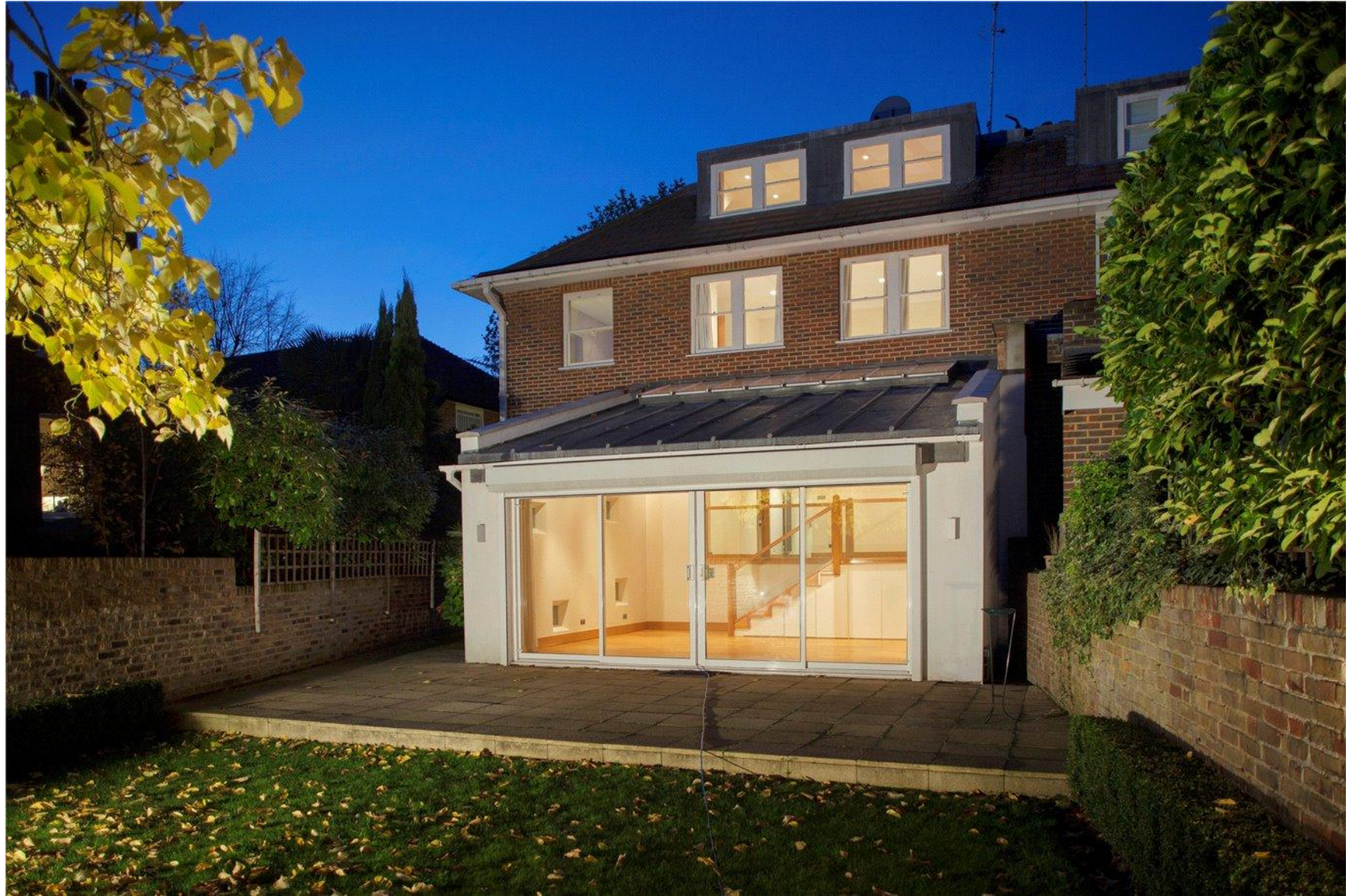
SPRINGFIELD ROAD 3 St John's Wood, NW8
