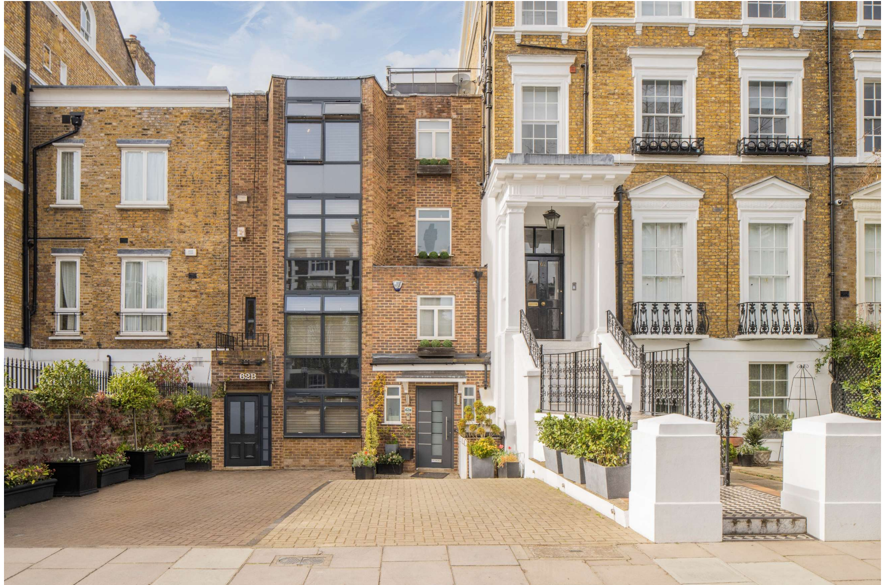
MARLBOROUGH PLACE St John's Wood, NW8
