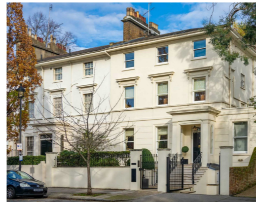
Cavendish Avenue (Grade II listed) | 5,500 sqft St John's Wood Conservation Area
