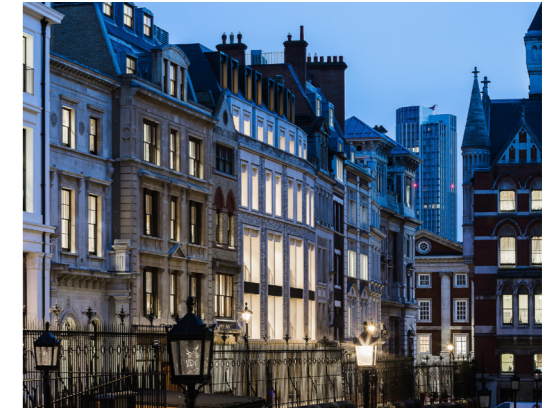
Bell Yard | 10,300 sqft The Strand Conservation Area
