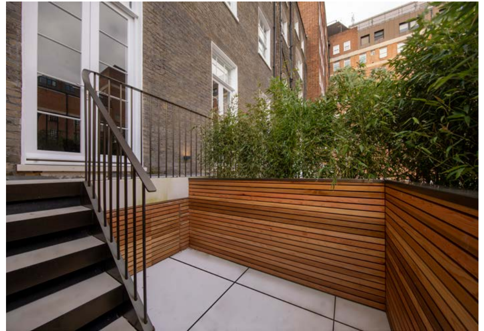
LEFT KITCHEN ABOVE PRIVATE CEDAR CLAD TERRACE
